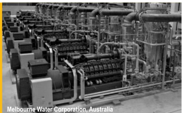
The plant can convert the emerging sewage gas to electricity so that the energy self-demand is covered. These gas gensets convert natural and sewage gas into 1.4 MW electricity each. The thermal output from Jacket Water and Exhaust gas accounts for 1.4 MW per engine as well.
