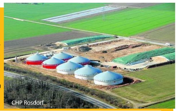
Adjecent to the tax office building of Goettingen the biogas plant Rosdorf, equipped with three gas engines CG132-12 rating of 600 kWe each. These are generating 25 million kWh of heat (Warm Water) annually, plus electricity for 5,000 homes by utilizing the biogas from the plant, fed by Biomass from the region.
